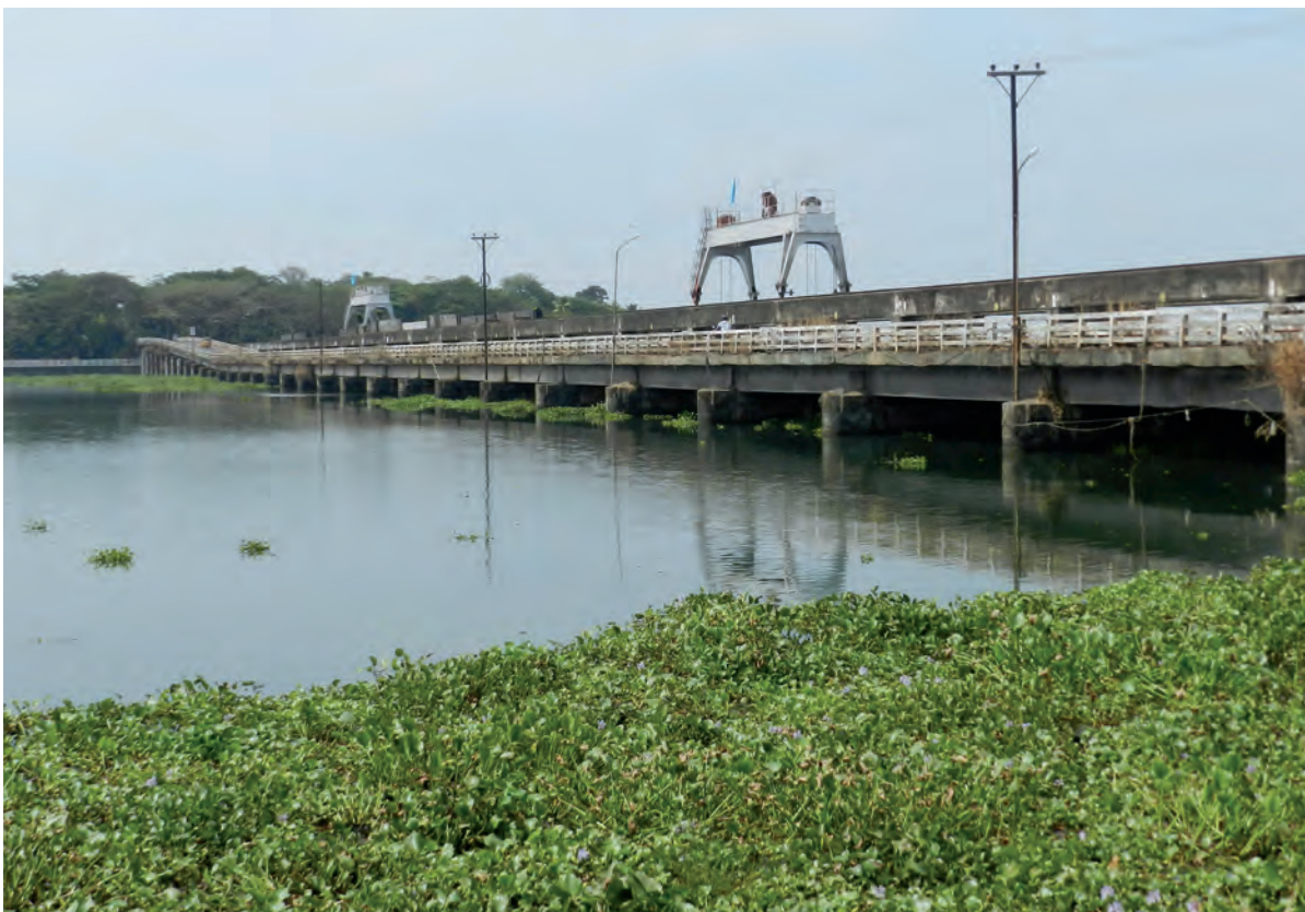
View of Thaneermukkom Barrage from southern end
